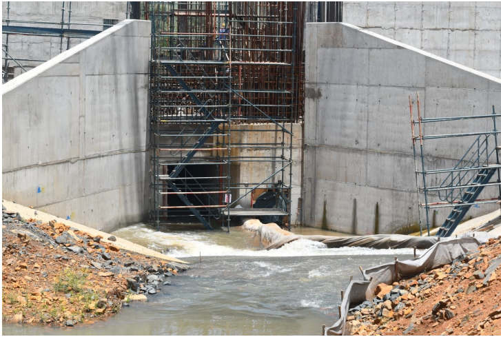
Under Construct: Gabosch Dam in Amsterdam in Ward 05
