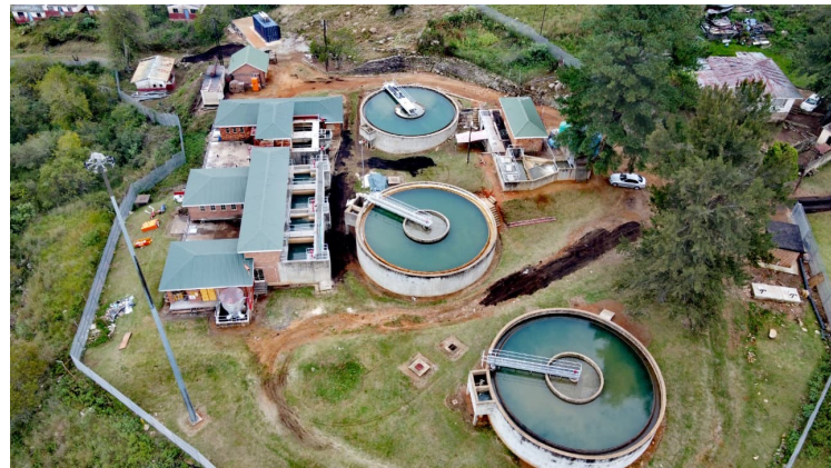
Newly Refurbished eMkhondo Water Treatment Plant.
